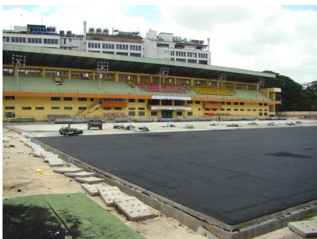
Figure 6: sub-base preparation for a FIFA Goal project in Greenland ©Greenfields
