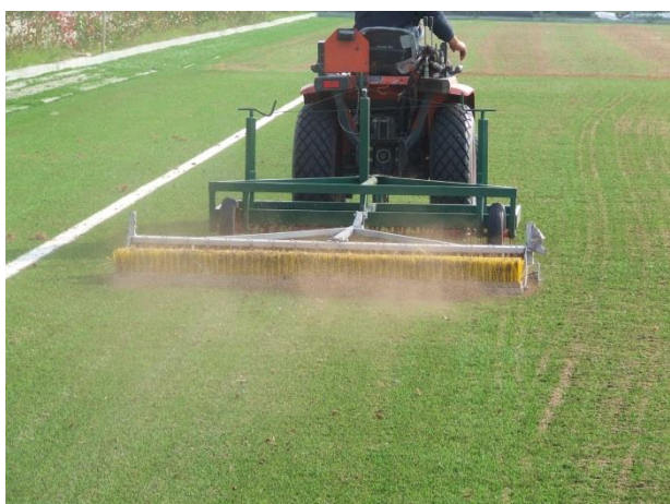
Figure 9: installation of the infill material ©Limonta
