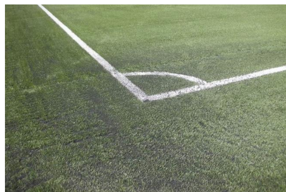
Figure 14: accumulated infill material in the corner area
