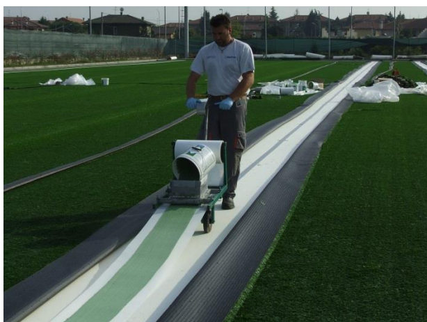
Figure 8: preparation of the seam tape ©Limonta
