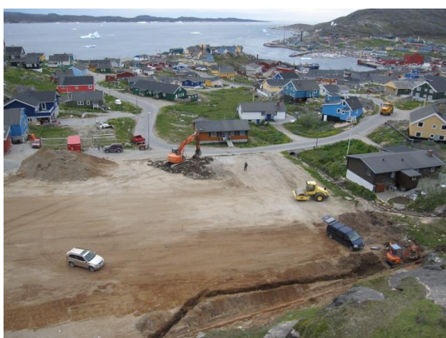
Figure 6: sub-base preparation for a FIFA Goal project in Greenland ©Greenfields
